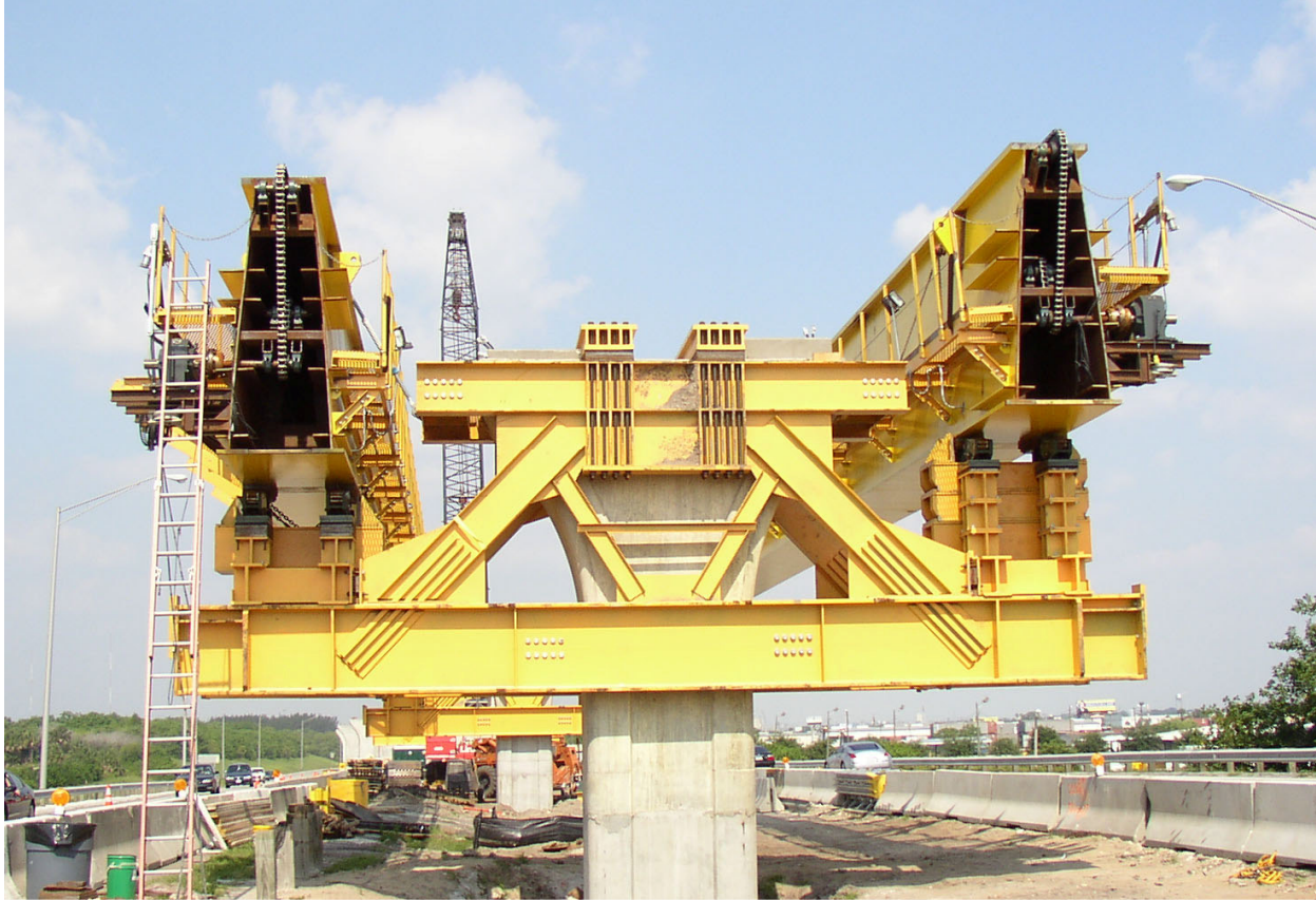
Photo 1: Pier Bracket and Erection Girders
