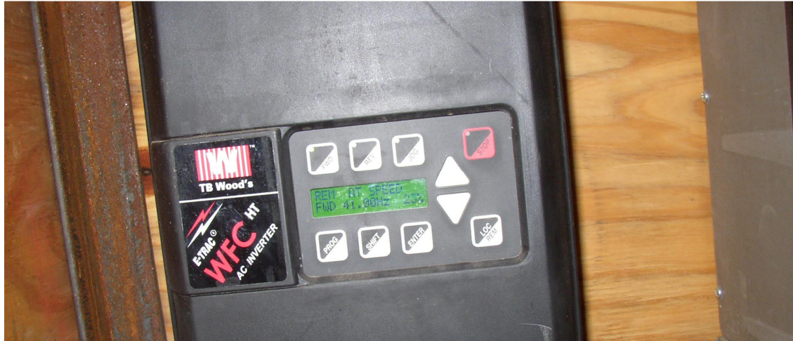
Photo 6: VFD at Load, 41 HZ or 15 feet per minute Note Load at 23% Plenty of Reserve Power
