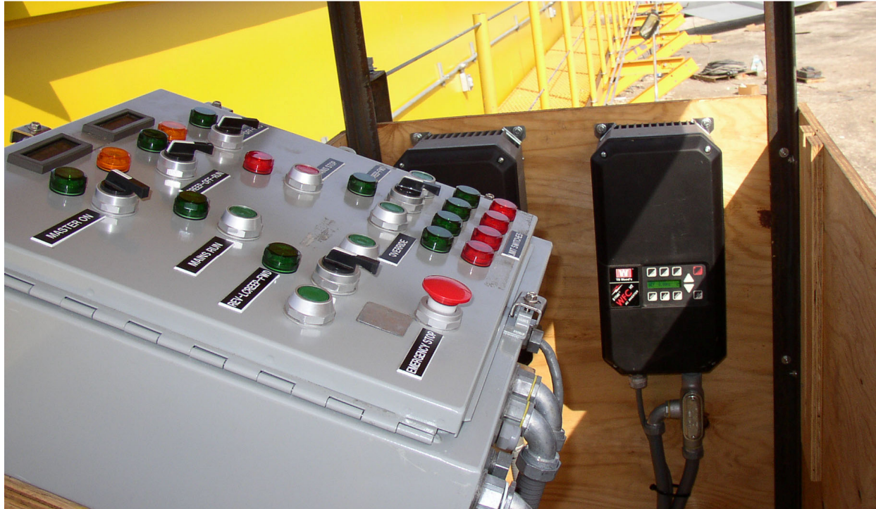
Photo 3: Control Panel, Heading One, VFDs Behind
